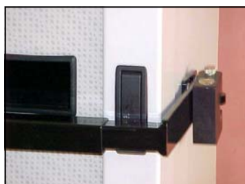
Door strap preventing unauthorised access
