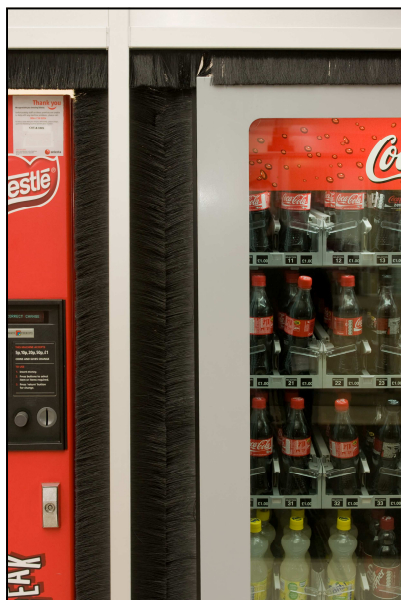
(Above) The brush strips provide a tidy finish, whilst allowing for access to the sides of the machine.
